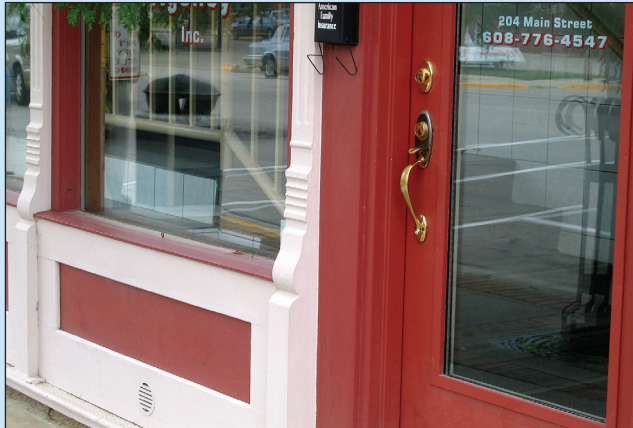
Figure 4-31. Businesses along Main Street in Darlington, WI, mitigated with an elevated interior first floor
