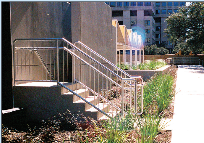
Figure 3-25. Three sets of stairs that provide building egress during the design flood event, but still allow normal use of the building (source: Walter P. Moore)
